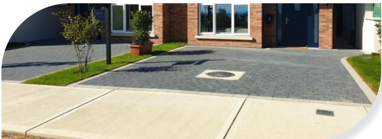
Figure 2.4: Permeable Paving Driveways to promote Infiltration
