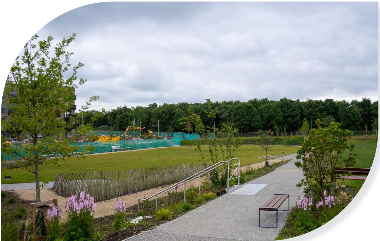
Figure 3.2: Detention Basin at Clonburris
