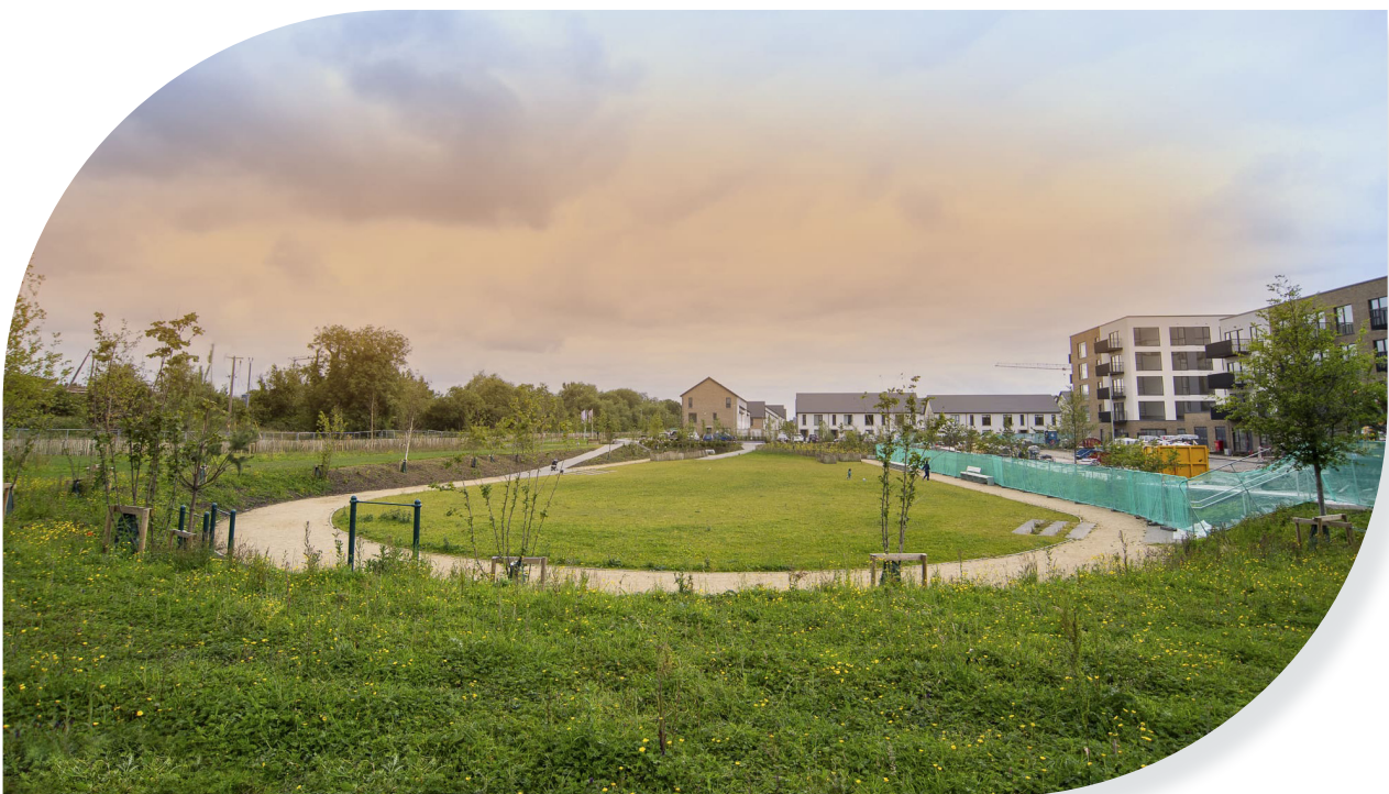
Figure 2.1: Detention Basin with Residential Development
