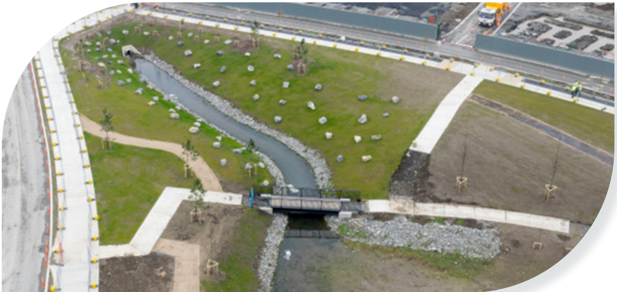
Figure 3.7: Drone Images of the Central Wetland under construction (Captured 17/02/2025)
