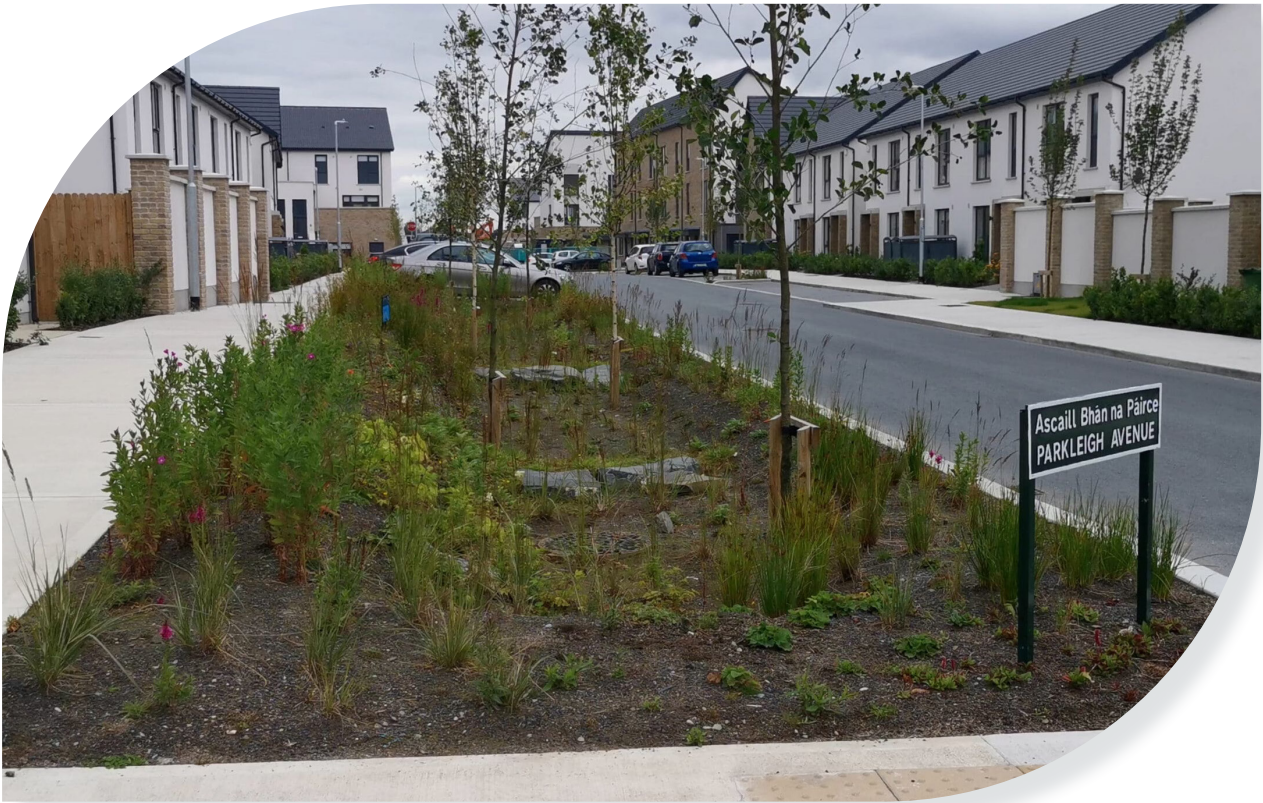
Figure 3.3: Bio Retention Area at Clonburris
